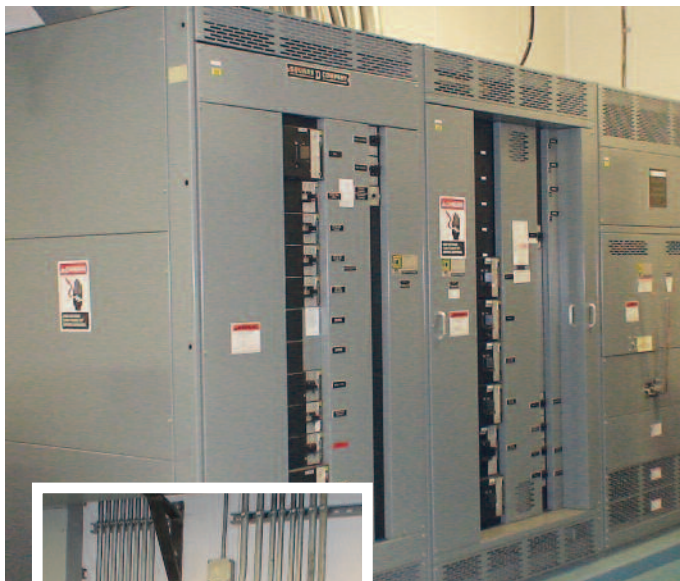
ABOVE: BEGINNING WITH THE MAIN SWITCH GEAR, THE SYSTEM FILTERS THE POWER FOR THE ENTIRE FACILITY. THIS INCLUDES LIGHTING PANELS, DRIVE CABINETS, MOTORS AND OTHER EQUIPMENT.
