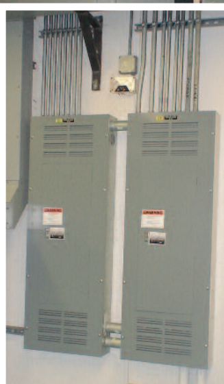
ABOVE: BEGINNING WITH THE MAIN SWITCH GEAR, THE SYSTEM FILTERS THE POWER FOR THE ENTIRE FACILITY. THIS INCLUDES LIGHTING PANELS, DRIVE CABINETS, MOTORS AND OTHER EQUIPMENT.
